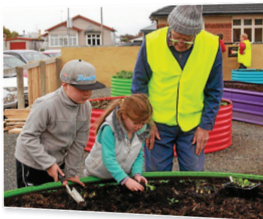
Above: Maurice Tucker and his grandchildren weeding one of the community garden boxes. Marie Crowe in the background building a garden box on top of the fence. The paling fence under construction on the left.
